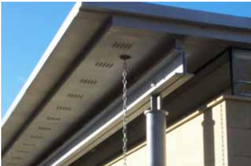
Aluminium Roof with chain rainwater downpipes
